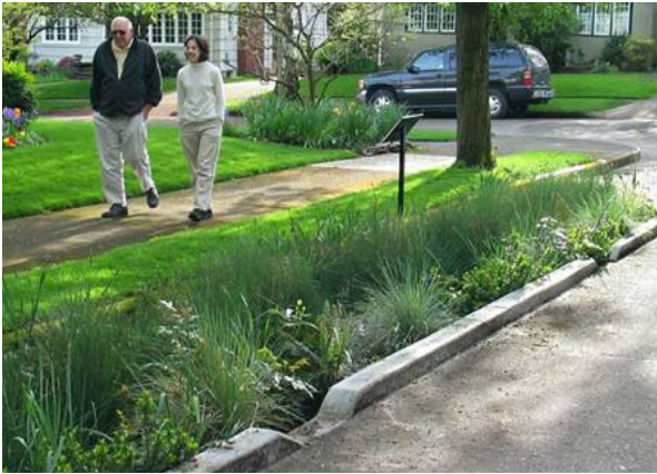
Example of Integrated Soft Landscape and Stormwater Treatment
