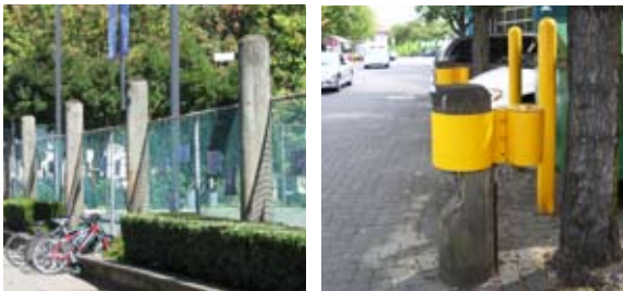
Awning/canopy supports, fencing and bollard components and service area enclosures integrate recycled wooden poles into the design
