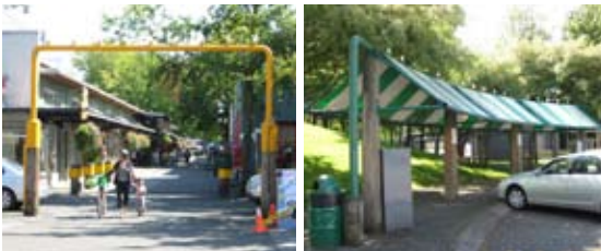
Recycled wooden poles integrated into parking lot structures and supports for awnings and signage
