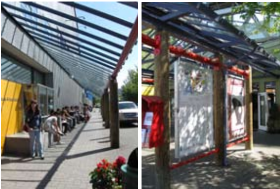
Recycled wooden poles integrated into parking lot structures and supports for awnings and signage
