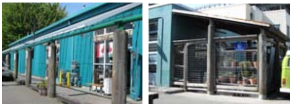
Awning/canopy supports, fencing and bollard components and service area enclosures integrate recycled wooden poles into the design
