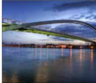
1. No. 2 Road Bridge
