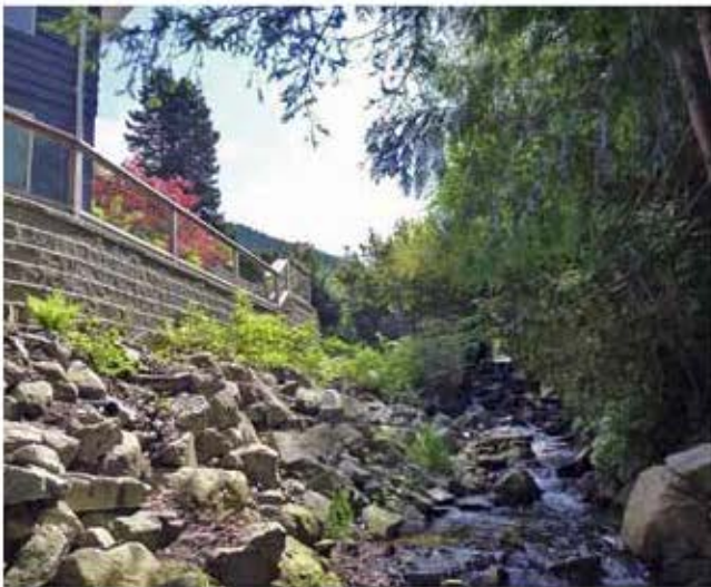
A new foundation and creek bank stabilization project, after the creek eroded the foundations of the existing house (left). Debris Flow risk reduction: Debris catch basin on one branch of MacKay Creek (right).
