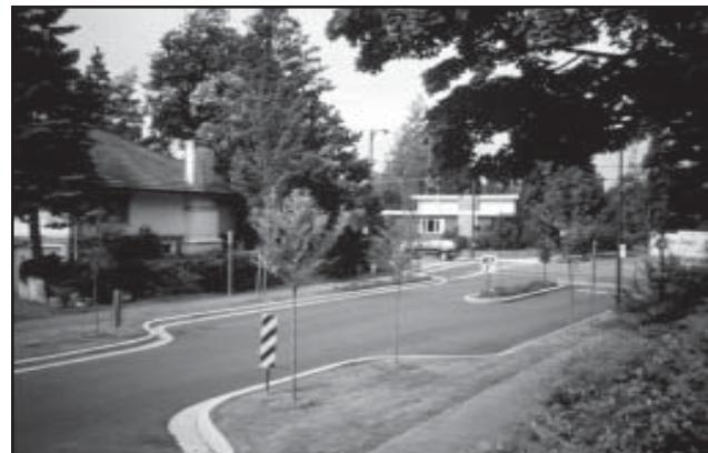
Where a high need to discourage through traffic has been demonstrated, maintain a continuous street grid for pedestrians, cyclists and emergency vehicles (e.g., through diverters and “right-in, right-out” devices).
