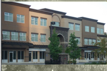
City Scape Building
