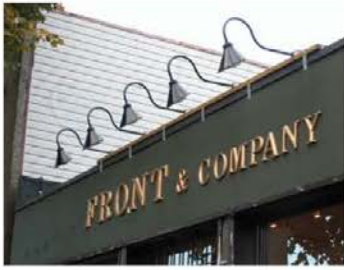
Figure 36. Down lighting with cutoff shields reduces glaring light sources.
