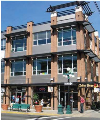
Figure 42. Fixed fins shade the interior from afternoon sun, reducing summer cooling loads
