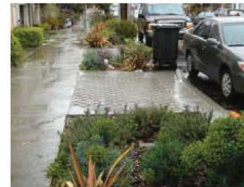
Figure 41. Storm water source controls like these rain gardens reduce pollutant run-off.
