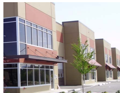
Where appropriate, all buildings should provide impression of two stories with the use of spandrel glass
