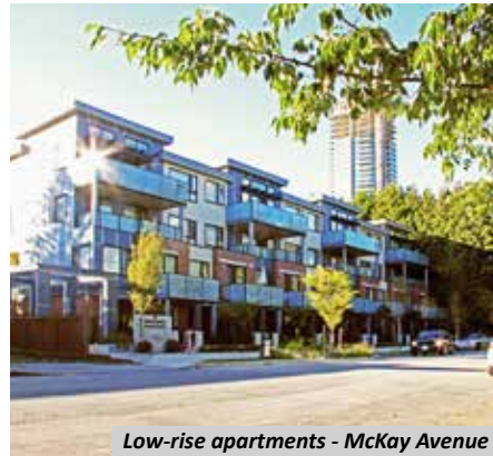
Low-rise apartments - McKay Avenue
