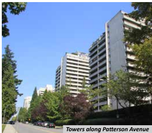
Towers along Patterson Avenue
