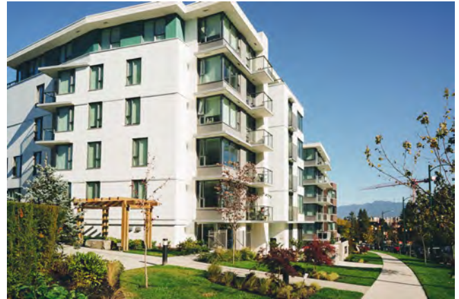
Figure 5.2: 6 storey arterial building
